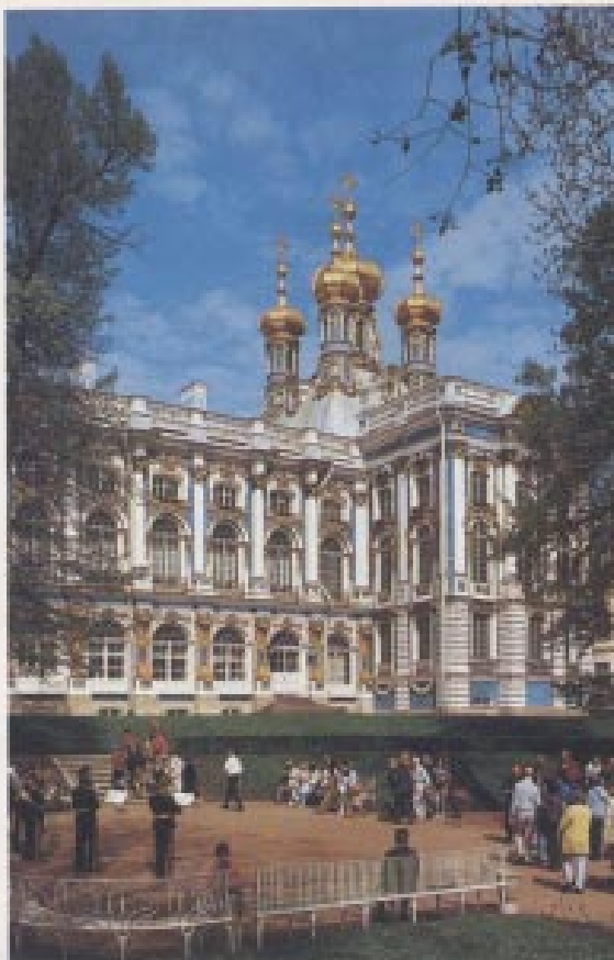
The main facade of Pushkin Palace © J. Woodhead
